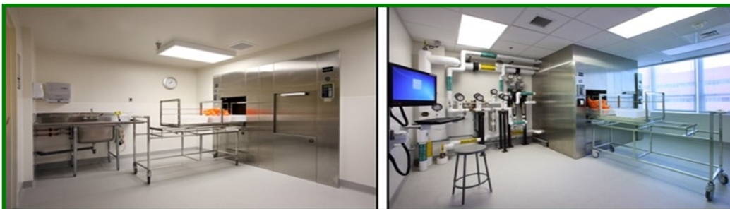
The dirty side (left panel) and clean side (right panel) of the Biocontainment Unit waste management area. The dirty side of the unit requires high-temperature autoclaving of all materials before removal. The clean side of the unit means all material passing through the autoclave may be safely handled.
