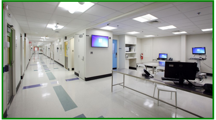
The Biocontainment Unit has completely separate ventilation systems from the rest of Johns Hopkins hospital, as well as strict entry/exit protocols to prevent spread of infection.
