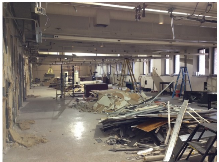
Demolition of the space designated for the Fisher Center
